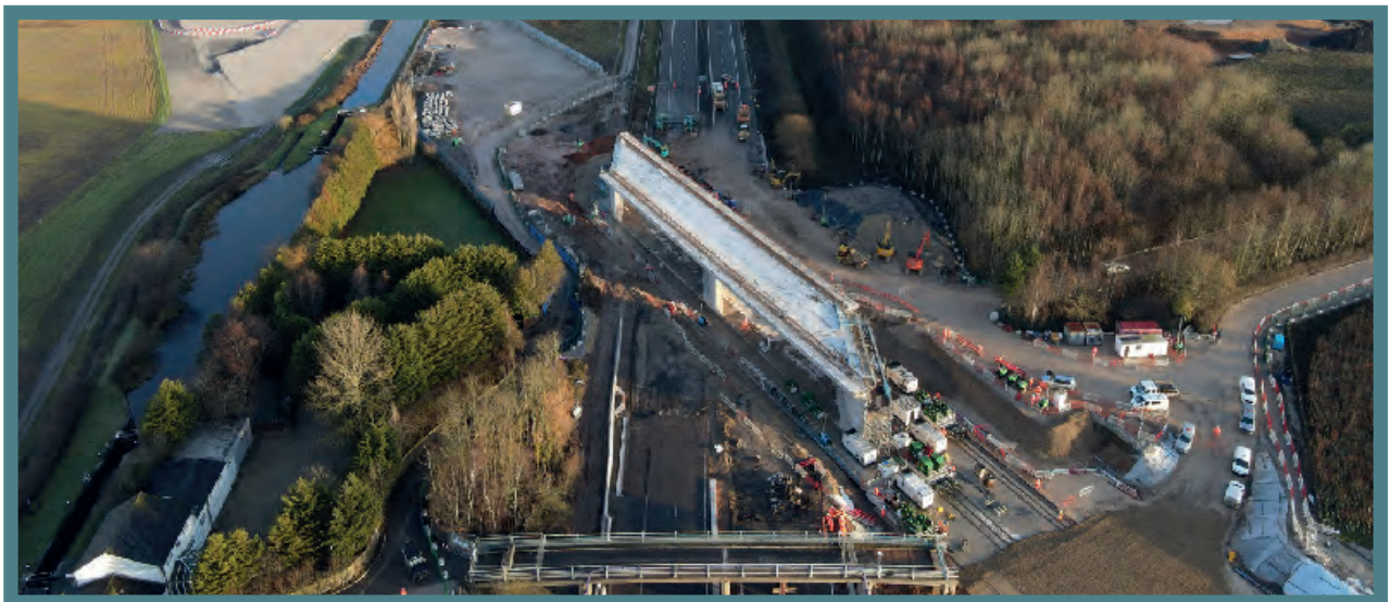
ABOVE: AN AERIAL OF THE WORLD'S LONGEST BOX BRIDGE SLIDE ACROSS THE M42.
