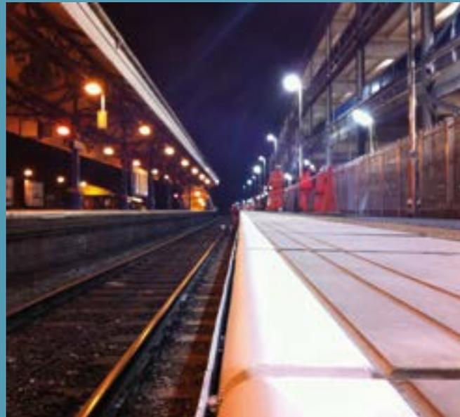
The front inserts are placed into transverse beams to approximately the correct gauge. A calibrated platform gauge is set up on track and set to the correct gauge (making allowance for fascia plate, deck pans and platform coper units).
