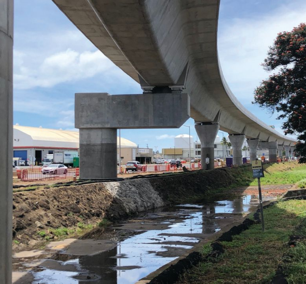
Figure 6. L-bents were used when there was limited access to place a pile cap. The most extreme case on the project occurred over the Aolele Canal, where there is a 17 ft offset between the center of the guideway and the column. Photo: SYSTRA International Bridge Technologies.
