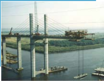
Fig. 21. Shown is the Neches River Bridge lifting segment in Texas.
