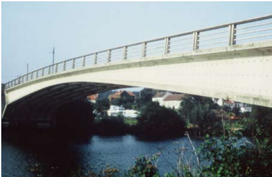
Fig. 3. Shown is the Esbly Bridge on the Marne River in France.
