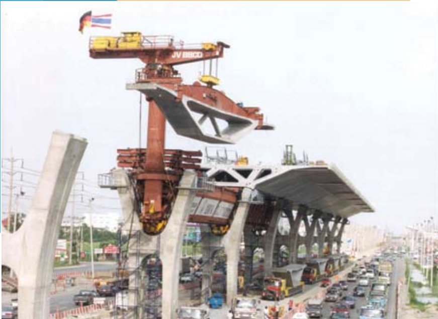
Fig. 24. Shown is the Bang Na Expressway in Bangkok, Thailand.
