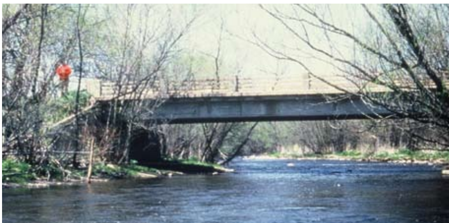
Fig. 4. Shown is the Shelton Bridge in upstate New York.
