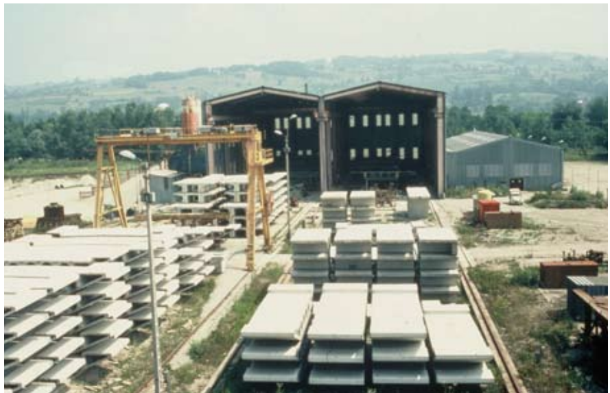
Fig. 11. Pictured is the Alpine Motorways precasting factory in France.
