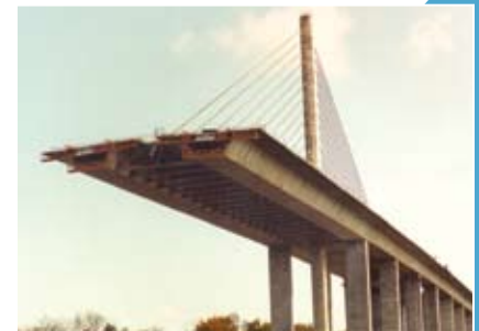
Fig. 19. The C&D Canal Bridge delta frame system photographed in Delaware.
