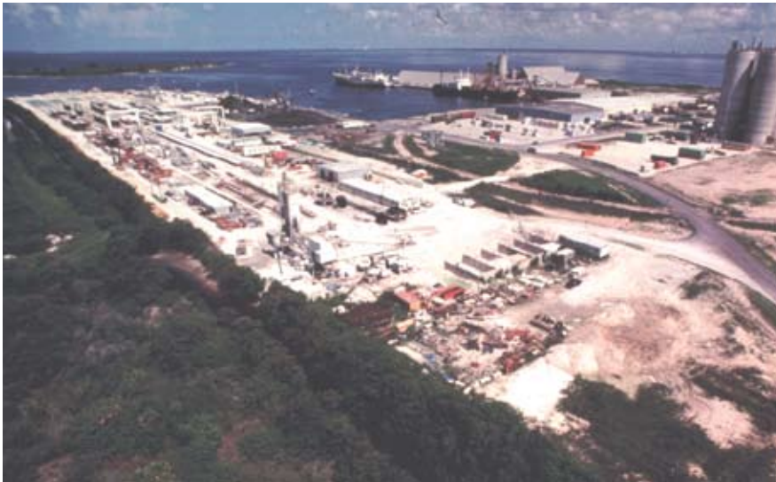
Fig. 18. Shown is the Sunshine Skyway Bridge precasting yard at Port Manatee, Fla.
