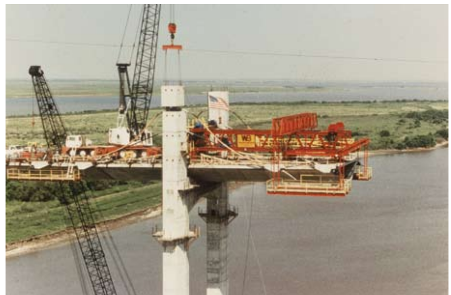
Fig. 20. Pictured is the Neches River Bridge precast concrete pylon in Texas.
