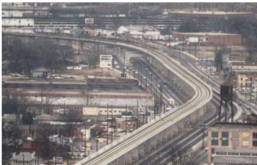
Fig. 16. Shown is the MARTA light rail viaduct in Atlanta, Ga.
