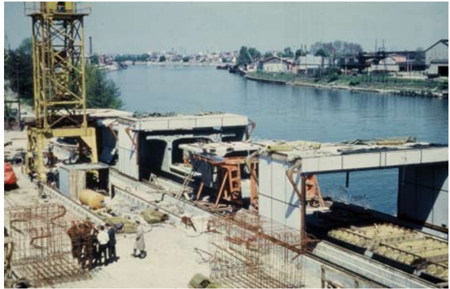
Fig. 7. Shown is the long-bed precasting at the Choisy-le-Roi site in Paris, France.
