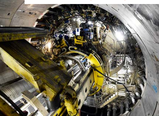
TUNNEL BORING MACHINE, TELT PROJECT, FRANCE-ITALY
